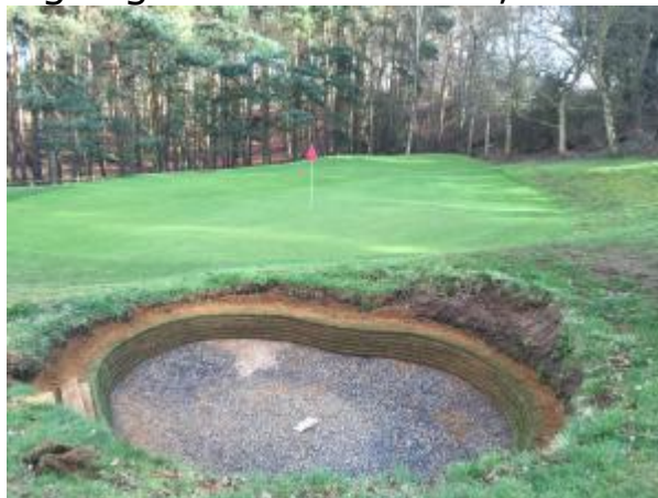
11th Hole, right green side bunker, work in progress.
